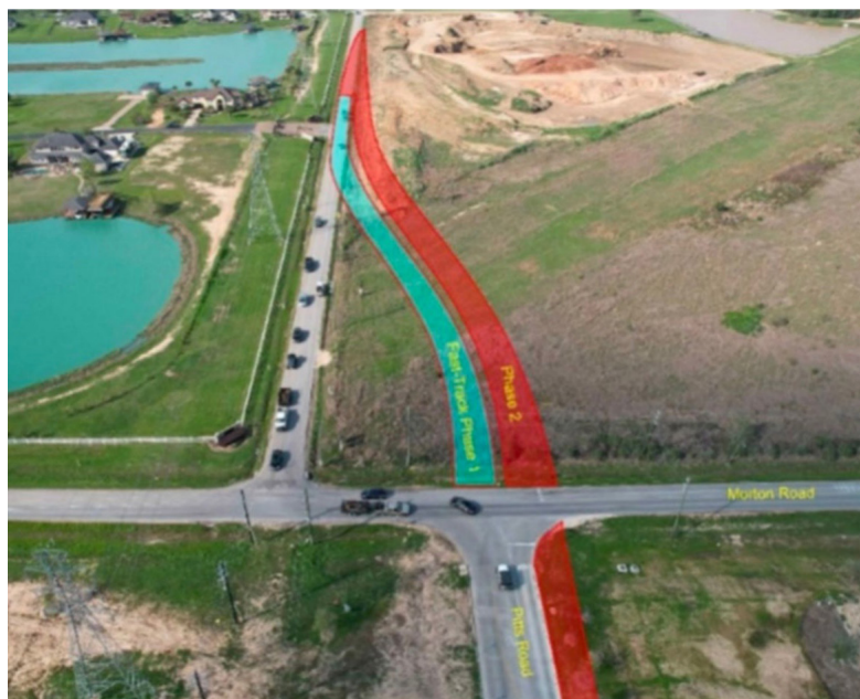
PHOTO TAKEN FROM ARKK ENGINEERING STATUS REPORT AND PROVIDED COURTESY OF COUNCILMEMBER DAN SMITH
