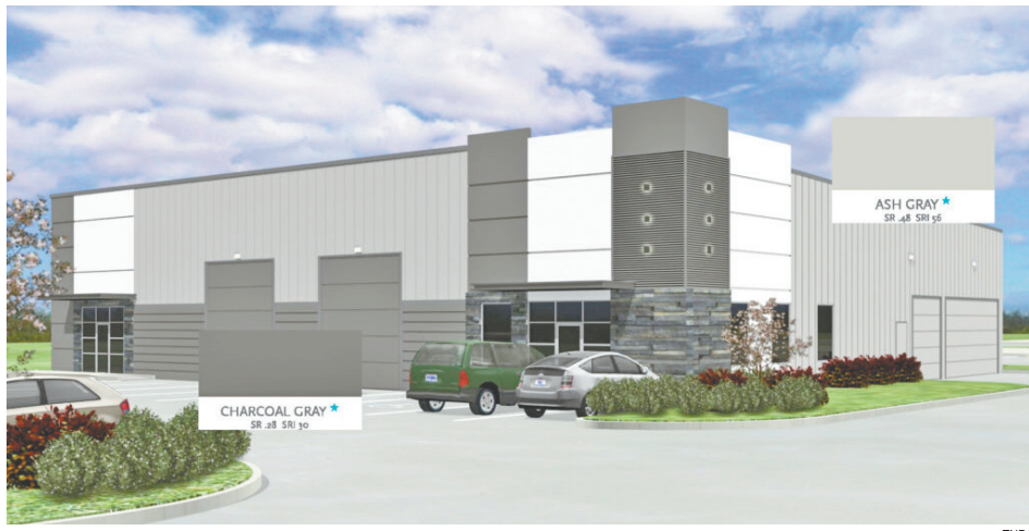
Buildings at the Katy Fort Bend Business Park will be colored in ash gray, peppercorn and extra white, as shown in this depiction. Buildings will feature 3' x 5' wall lite panels to allow natural light.
